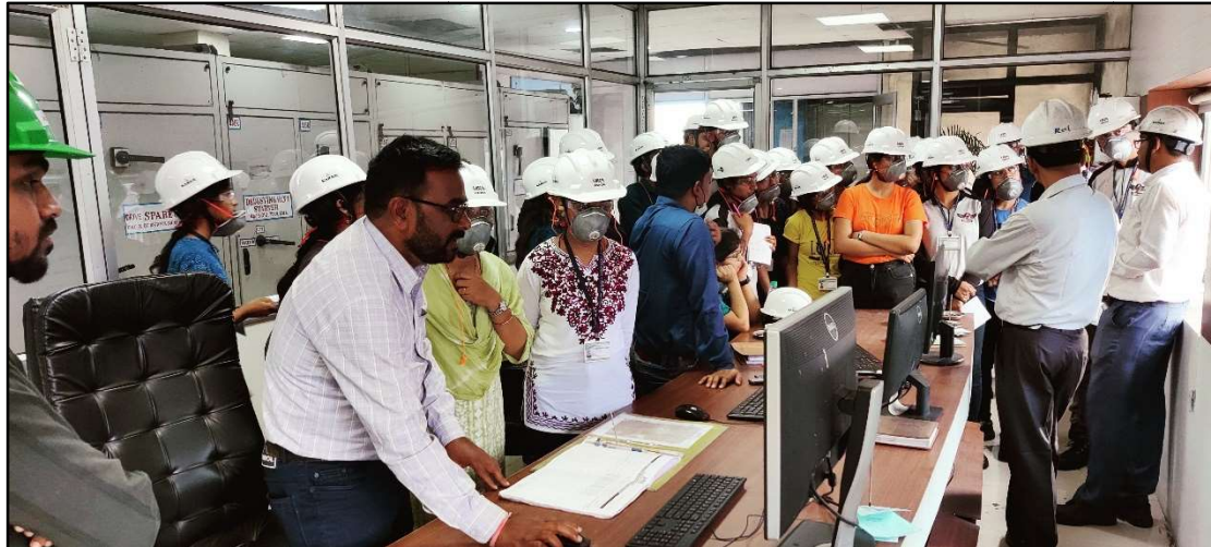
Inside the control room at Sponge Iron Division (SID)
